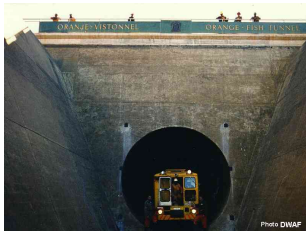
(a) Orange-Fish tunnel
