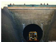
The Orange-Fish Tunnel (in Canada)
