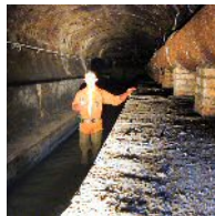
a sewer in Paris
